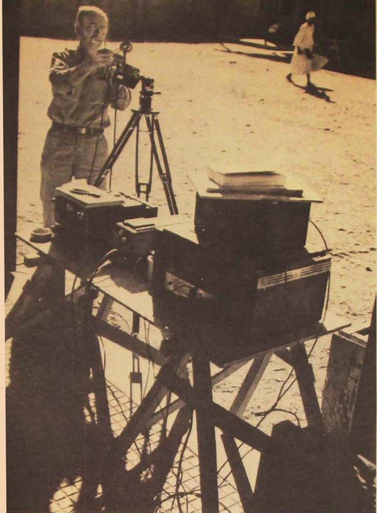
*Hundreds of hours were spent, both in the United States and in observation camps, training for the day of total eclipse. Here one of the scientists is testing his photoelectric cell and astrocompass. The device extending upward from the photoelectric cell simulates the various degrees of light variation during eclipse.*
