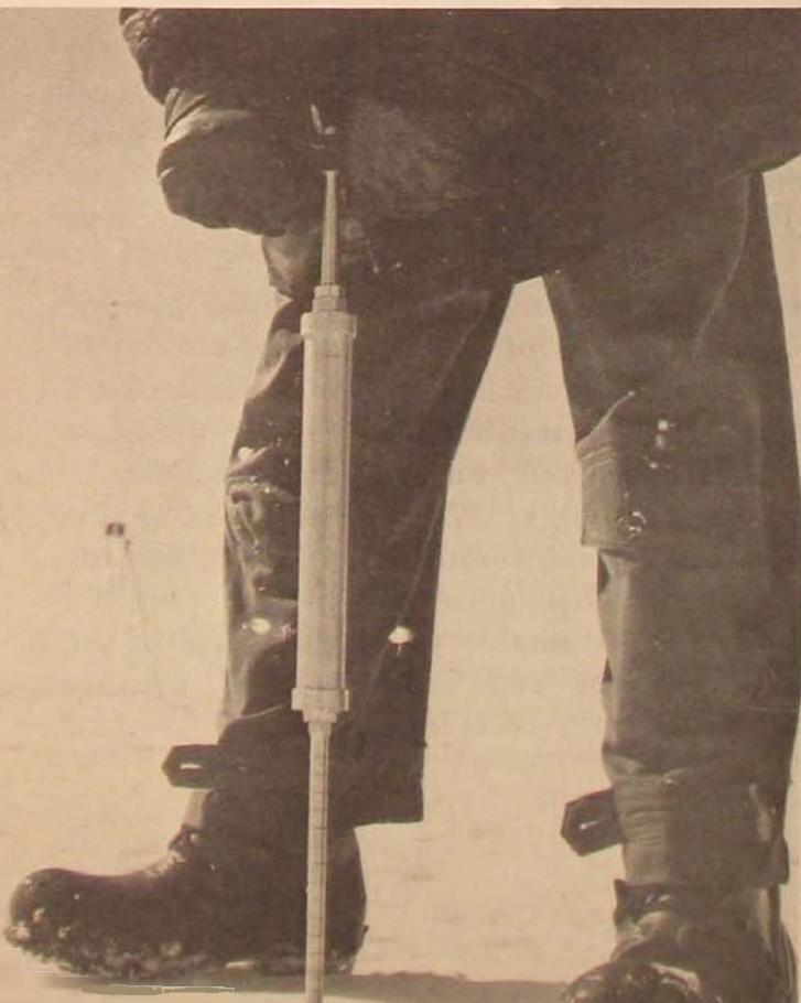
*A power drill that bored deep brought samples of various strata of ice to the surface for study. In certain areas drilling below a shallow surface layer of weak ice revealed basal ice strong enough to support any USAF aircraft.*
