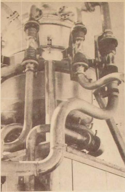
*Figure 2. Kiwi-A nuclear-rocket test reactor.*
