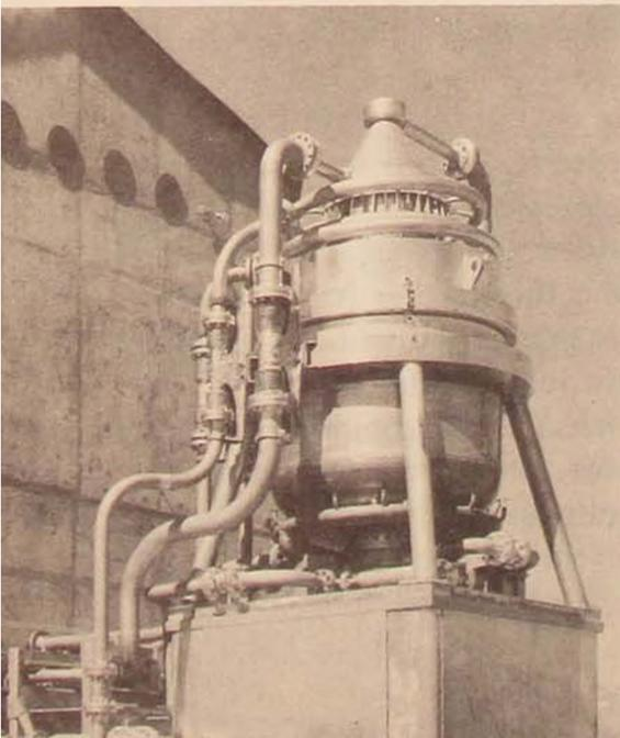
*Figure 2. Kiwi-A mockup positioned before test cell for alignment of water and propellant fittings. The reactor itself is in the large cylindrical pressure shell and is mounted on a cubical chamber that contains control and instrumentation gear. Supply lines plug into the face of the test cell at left. During the testing operations the reactor car is supported on outrigger rails.*
