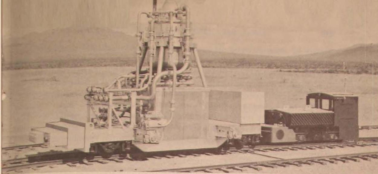
*Figure 3. The Kiwi-A mockup, mounted on its test car, being moved by rail from the MAD area to the reactor test area by the radio-controlled electric locomotive. The concrete umbilical plug on the nose of the test car carries the control and instrumentation lines and fits into an opening in the face of the test cell. The locomotive is removed from the test area during operation of the reactor.*
