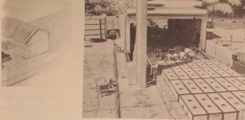
*Figure 1. Cutaway of NARF ground-test reactor shows (1) rail-borne concrete-block shield (also in photo above) that covers the pit when reactor is operating, (2) reactor pit, and (3) escalator system for lowering test items into position near the reactor. View down into the 3-megawatt reactor (right) shows fuel-element control rods and channels, gridded fuel-element cells, and remaining holes in grid-plate for additional fuel elements needed to make a critical mass.*
