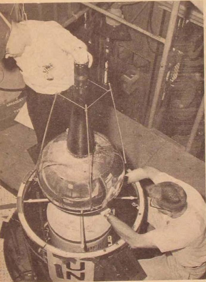
*Spread before the Vanguard III shell and magnetometer tube (above) are battery packs, electronics for space experiments, and transmitters. This last satellite in the Vanguard series is mated (left) to a Vanguard launching rocket, modified by NASA.*
