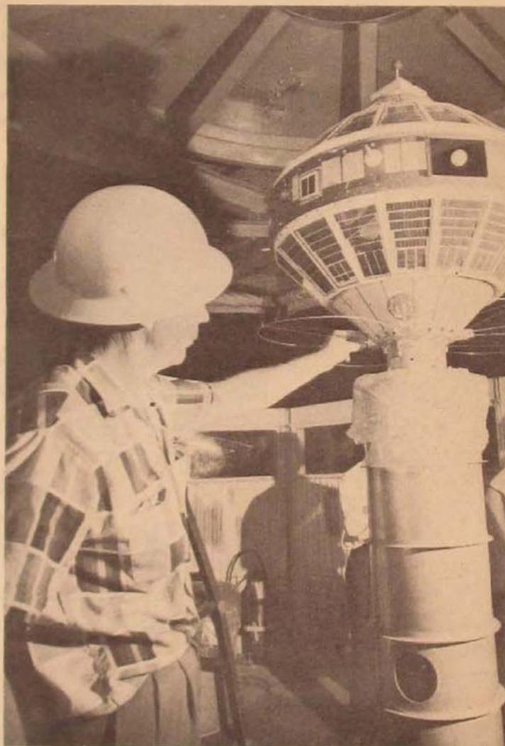
*Explorer VII, the composite radiation satellite and last IGY shot, undergoes final prelaunch inspection (right). The partially disassembled Explorer VII (top) and its 108-megacycle transmitter (above) show miniaturization of components.*
