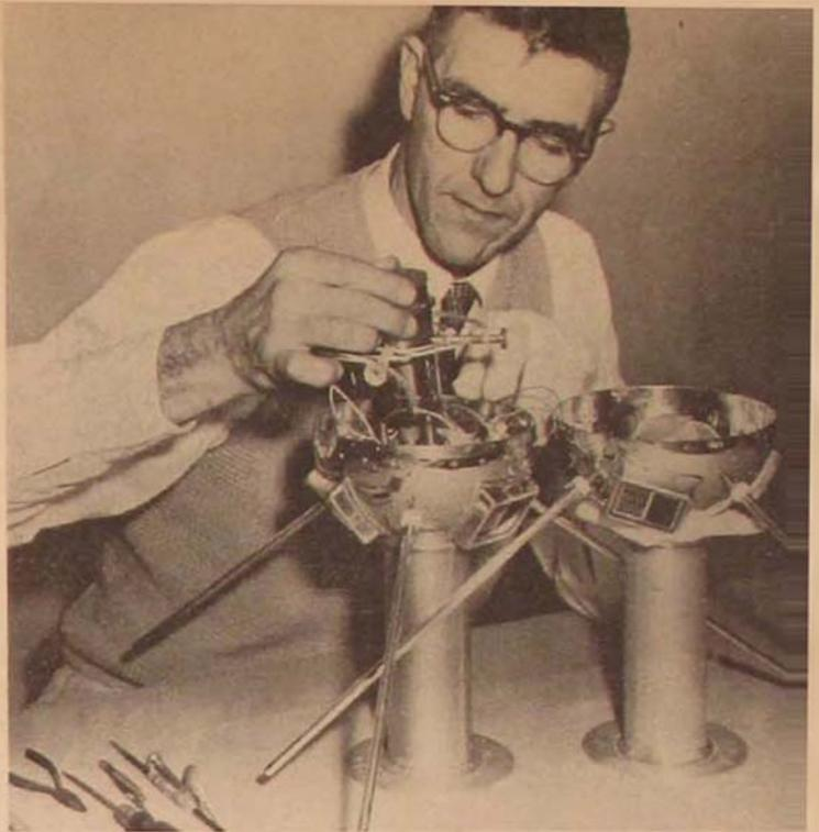
*Instruments are inserted in Vanguard I (above). Antennas and solar cells are on the satellite (left).*
