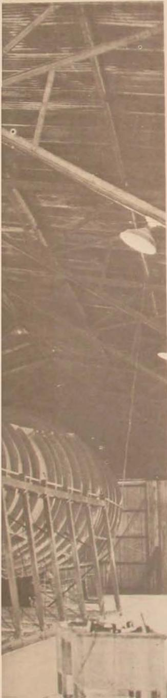
*Wind tunnel at McCook Field, 1922. Five feet in diameter and 96 feet long, the tunnel required the exclusive use of a 140-foot hangar. Scale models of airplanes, dirigibles, wings, etc., were mounted in the tunnel, and effects of the airstream on the model were measured. A 1/70 scale model of the triplane Barling bomber was among early aircraft that underwent tests in this tunnel.*
