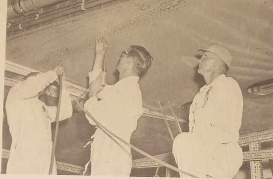
*Curing metal fatigue in the KC-135. Old method (above) required 8 days and 1600 man-hours. A locally designed pneumatic router mounted on a pantograph (right) reduced installation costs, cut flow time, and also ensured a job of higher quality.*
