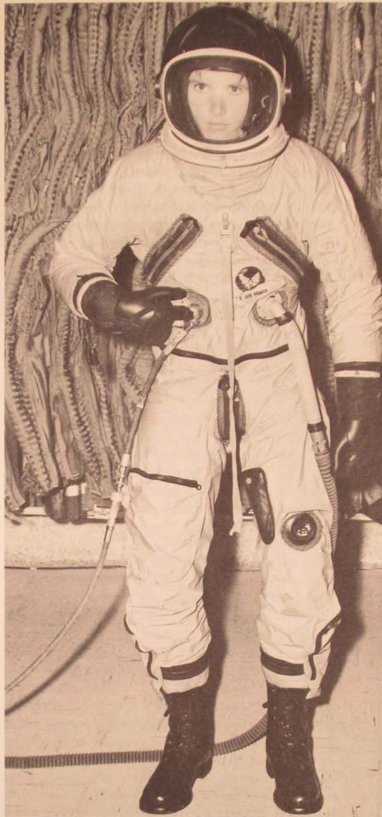
In 1962 the A/P22S-2, adapted from the Navy's Mark IV, became the Air Force's most advanced full pressure suit. Easy to put on and off, it ensures survival in water as well as at high altitudes.
