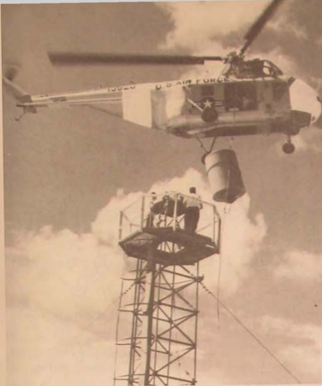
H-19 simplifies installation of tactical air navigation antenna.
