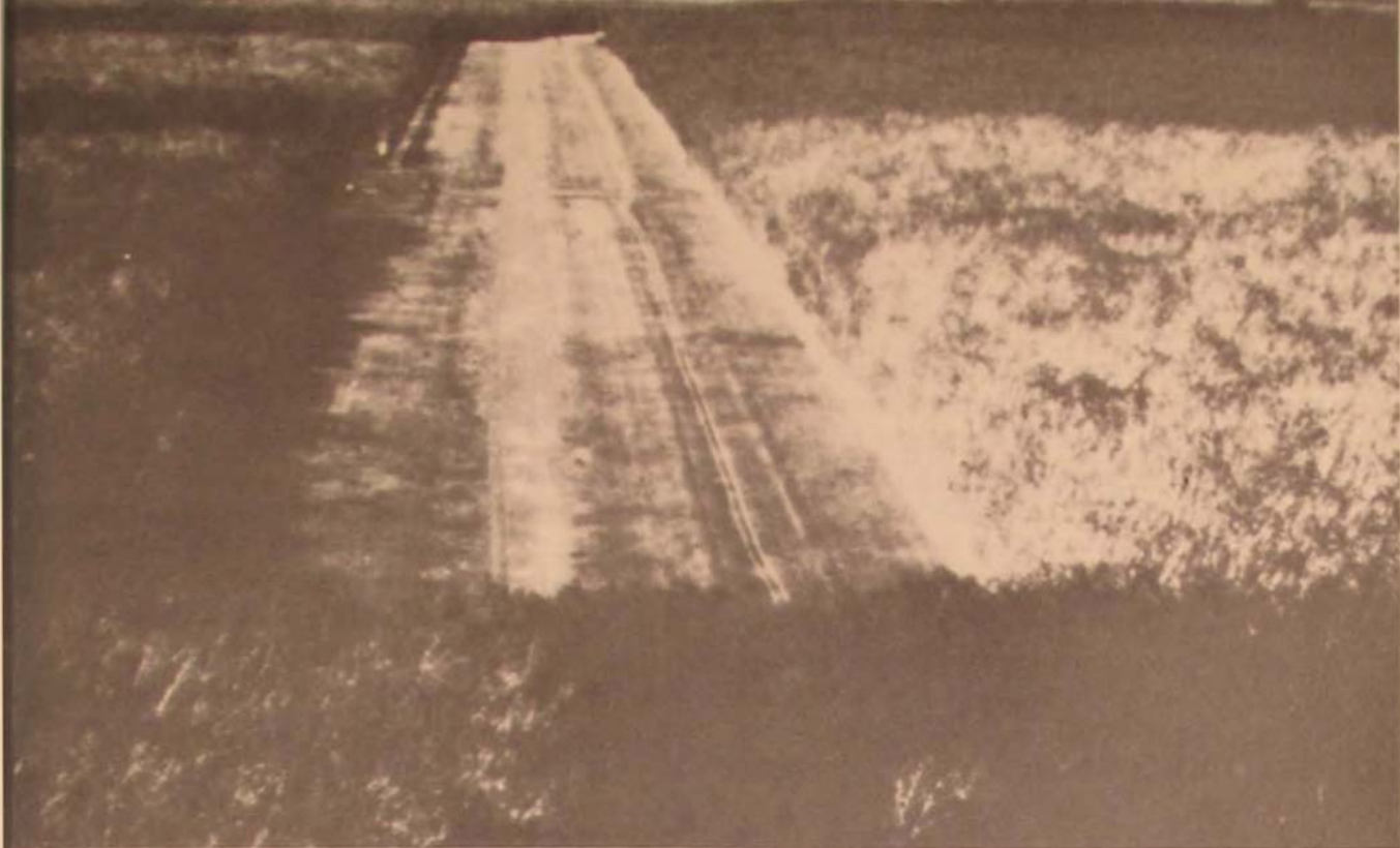
An airstrip that formerly served an old French plantation near Minh Thang is surrounded by rubber trees 200 feet high. Only 35 feet of the width of the strip can bear the load.
