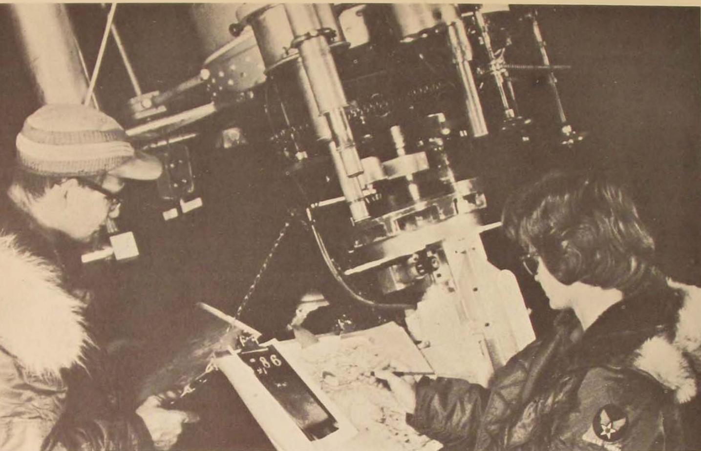
*At Lowell Observatory, Flagstaff, Arizona, (above) ACIC selenographers use large telescopes to identify minute lunar features. . . . Photogrammetric technicians skillfully match many lunar photographs to construct a composite photographic picture of the moon.*
