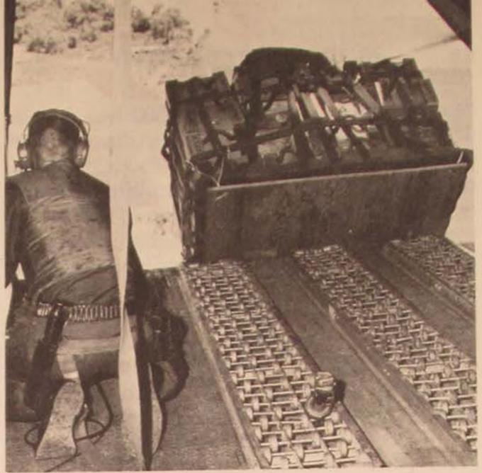
*Roller conveyer facilitates drop of palletized cargo.*
