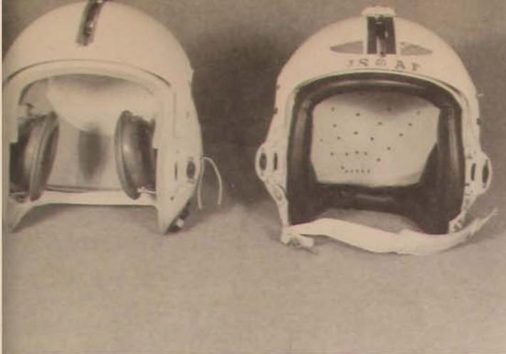
Compared to the standard issue helmet, the AFML custom helmet fits better, has only four inside pieces, and weighs less. . . . The photomicrograph (below) shows fiber orientation in a composite material reinforced with boron/epoxy tape. The boron fibers do not touch because better composite properties are thus obtained.
