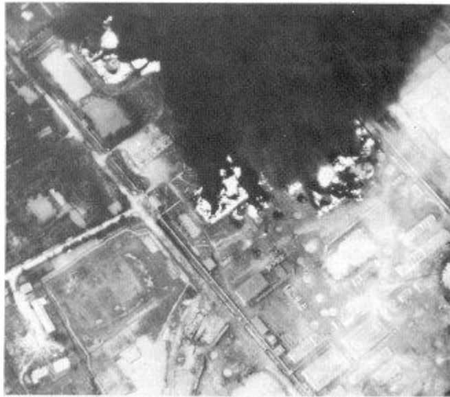
Hanoi Petroleum storage site. On 30 June 1966 Air Force F-105s bombed a petroleum storage area three miles north of Hanoi, North Vietnam. Although damage assessments indicated that the North Vietnamese petroleum storage capacity was 70% destroyed during Phase II of Rolling Thunder, destruction of such facilities had little impact on their ability to prosecute the war inside South Vietnam. 15
