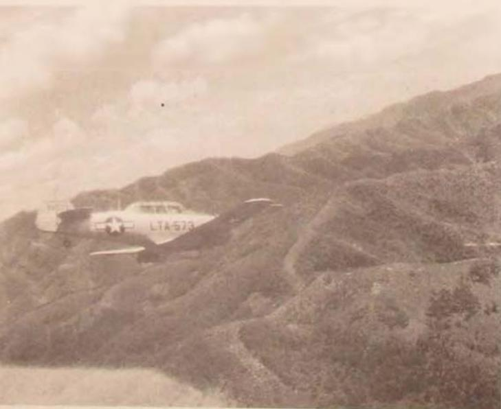
*The T-6 Mosquito forward air control aircraft was the mainstay of CAS air operations. Unfortunately, its limited communications and its vulnerability to ground fire hampered its effectiveness.*
