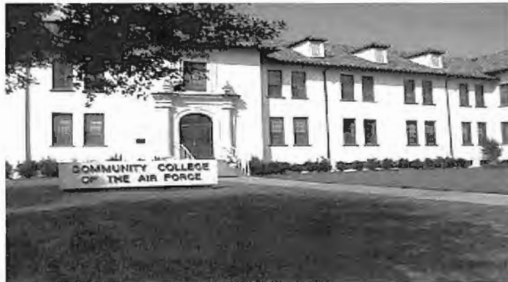
Simler Hall, CCAF Administrative Center Oldest building on Maxwell AFB—constructed in 1928
